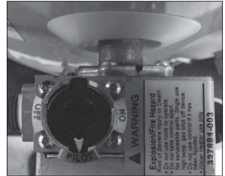
Figure 33 - Gas control/valve top view.
