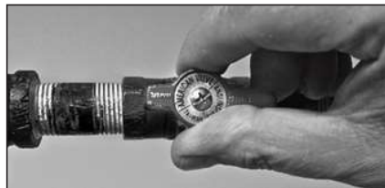
Figure 31 - Gas valve in "on" position
