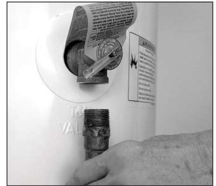
Figure 21 - Removing the T&P Relief Valve discharge pipe.
