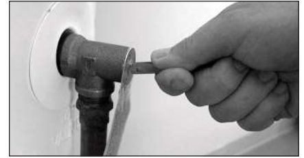
Figure 44 - T&P Relief Valve.
