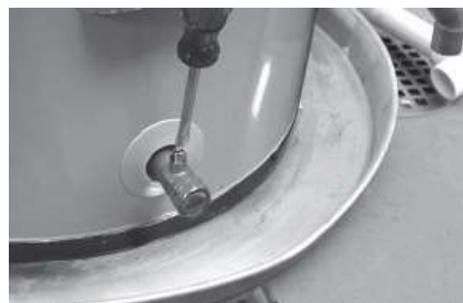
Figure 20 - Draining the old water heater.
