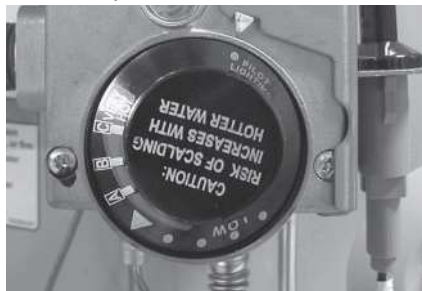
Figure 32 - Gas control/valve in Pilot Lighting position.
