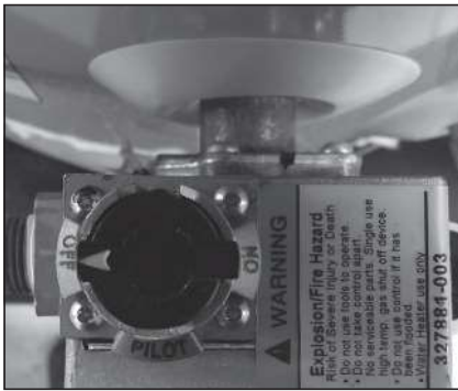
Figure 37 - Turn gas control knob OFF.
