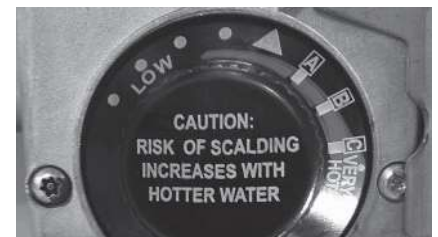
Figure 36 - Adjust the gas control knob to "▲".
