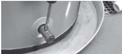
Figure 39 - Draining the water heater.
